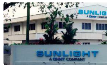
Sunlight Singapore & Malaysia Main Products: Low-voltage Switchgears
